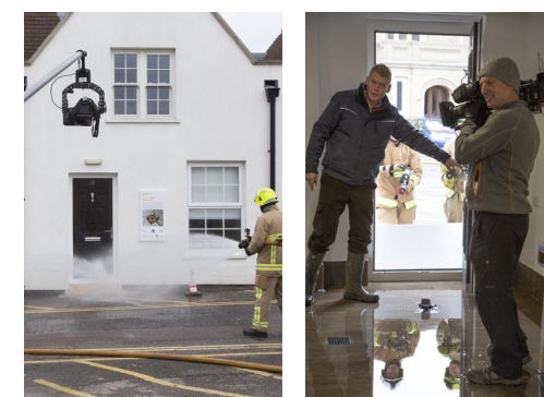
Flood Resilient Repair Home Watford, Angleterre, par Building Research Establish (BRE) / Photographies © BRE Group
